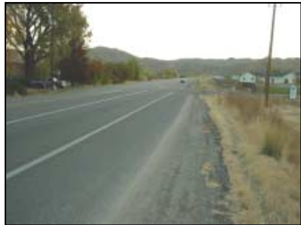
SH-16 West of Substation Road Looking East
